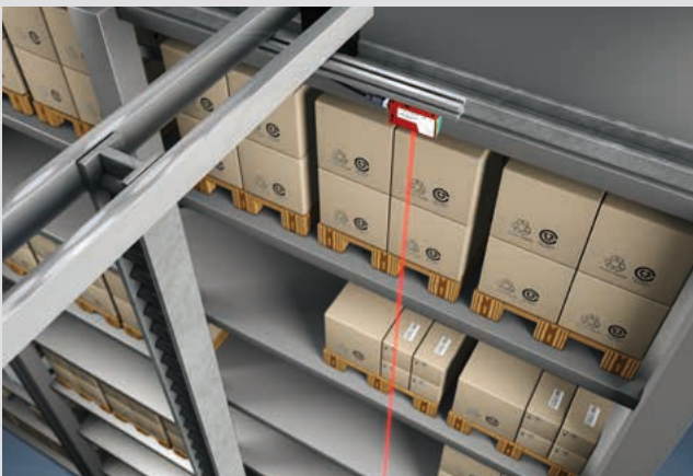
Gap monitoring on high-bay storage device
